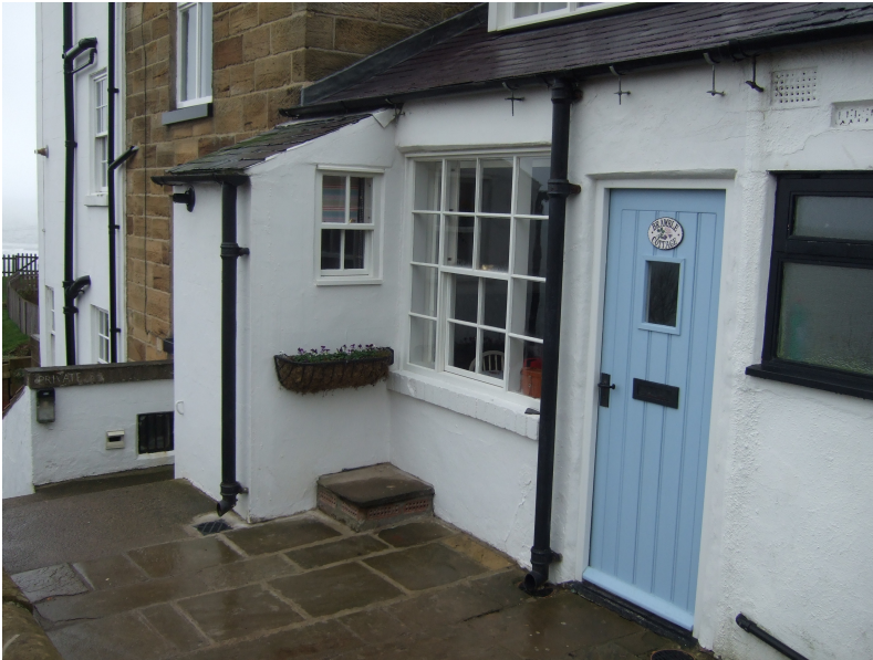
'Whitby Composite' windows - Robin Hood's Bay
