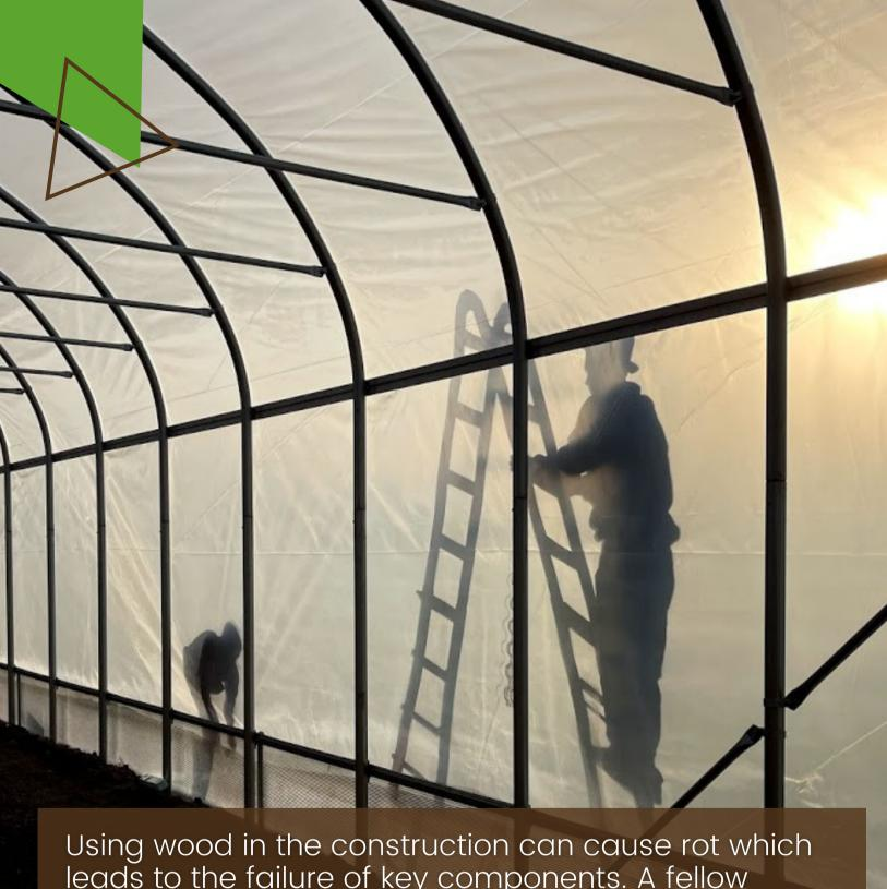
Using wood in the construction can cause rot which leads to the failure of key components. A fellow grower used wood hipboards on his tunnel to hold on the plastic. One cold January, a wind storm came up, the rotting wood gave way, and the grower lost an entire tunnel of greens. Building the entire structure out of steel and plastic is key for a long lasting, strong house.
