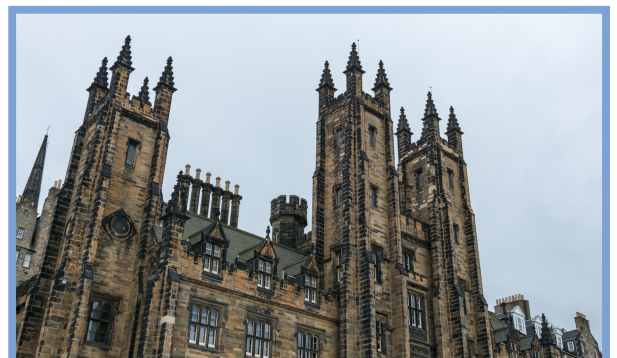
The Assembly Hall: the headquarters of the Church of Scotland.
